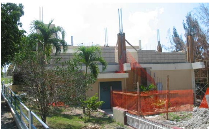
Construction begins on new CCRI facilities
