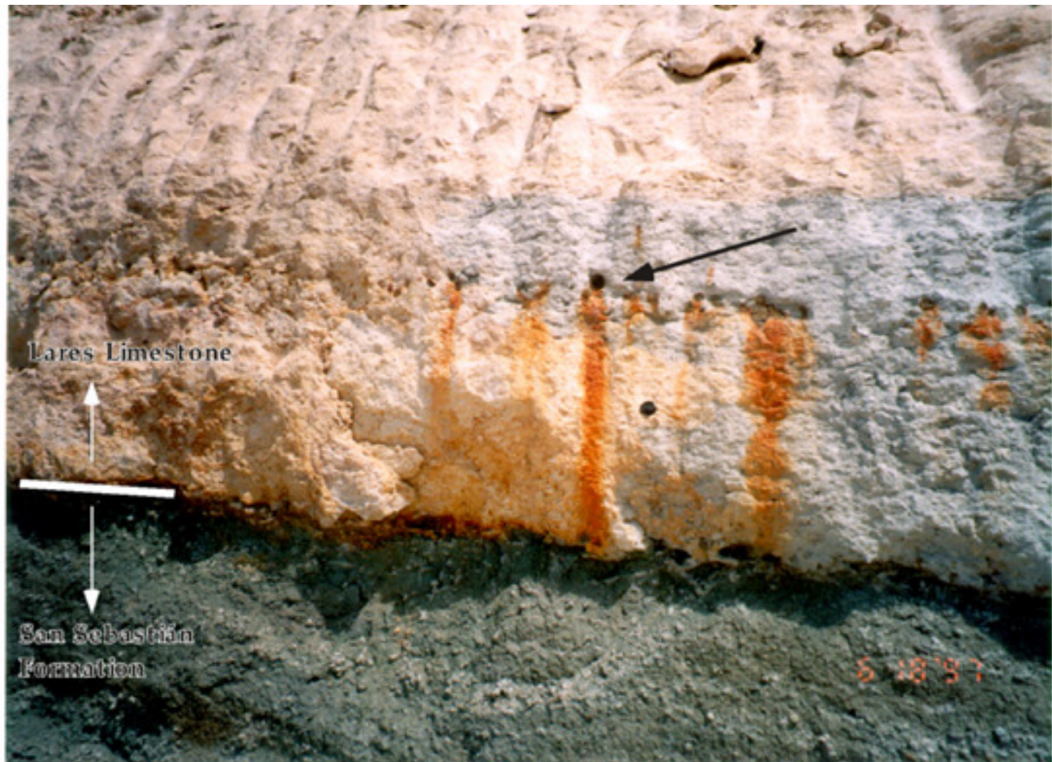
Fig. 8: The base of the Lares Limestone and its contact with the San Sebastián Formation exposed at the PR10-PR6621 intersection. Lines of cobbles composed of weathered (oxidized) volcanic rocks follow the apparent dip of the strata.
