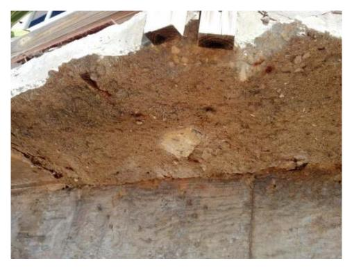
A4: Concrete wall erotion. Photo: P. Mejías.
