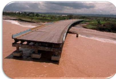
Figure 2 Víctor Rojas bridge was torn out of its foundation by a combination of storm surge and floodplain inundation caused by Hurricane Georges in September 1998. Credit to PrimeraHora and GFR Media.
