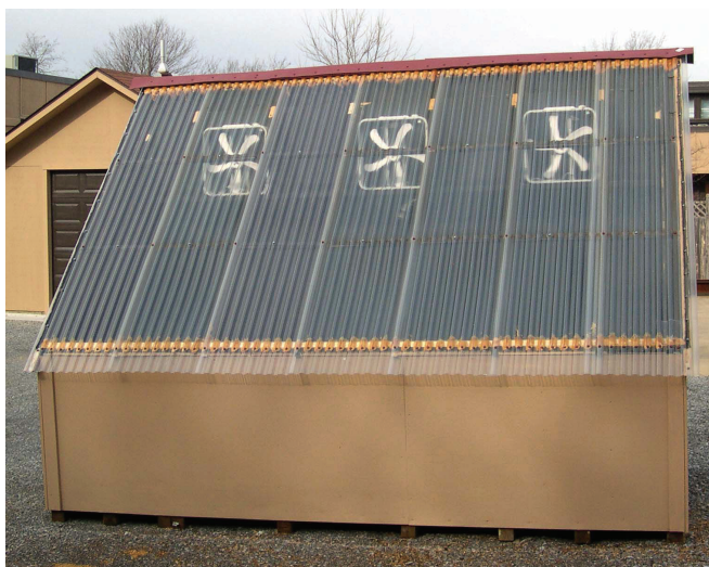
Figure 5—Front view of kiln showing fan placement.
