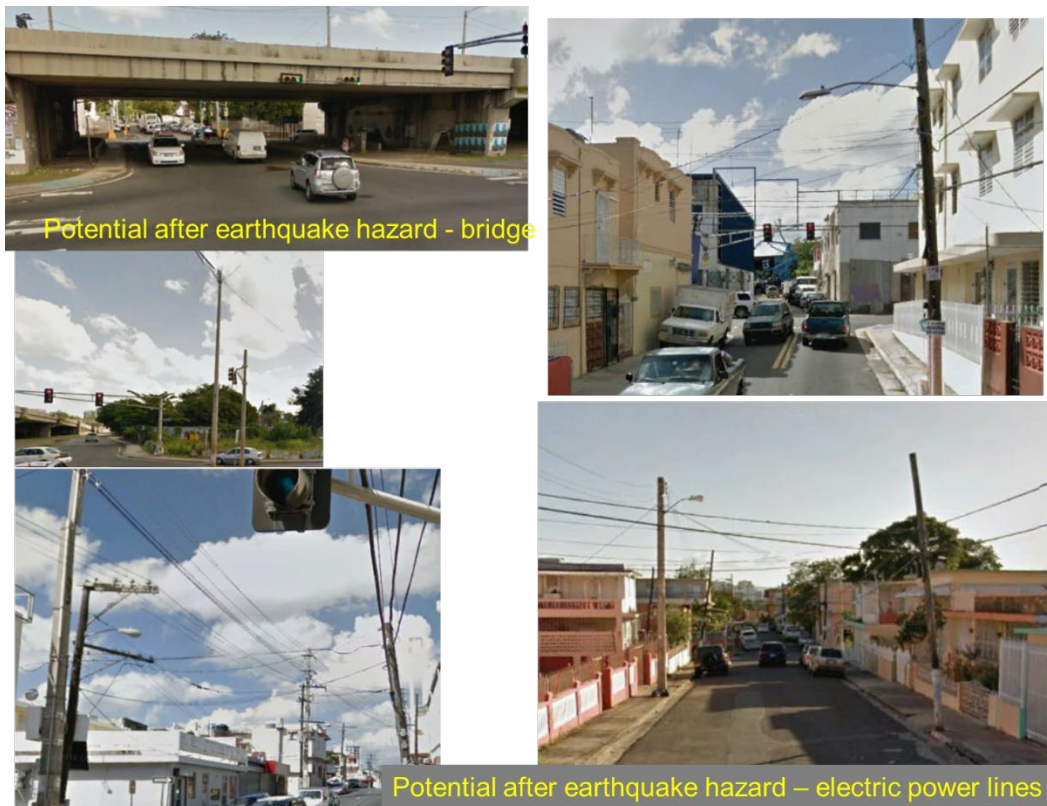
Figure 19: Obstruction on the Sidewalk and Potential After Earthquake Hazards for Luis Llorens Torres Evacuation Route.
