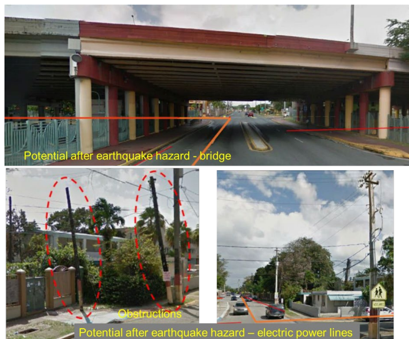
Figure 17: Obstruction on the Sidewalk and Potential After Earthquake Hazards for Francisco Oller Evacuation Route.
